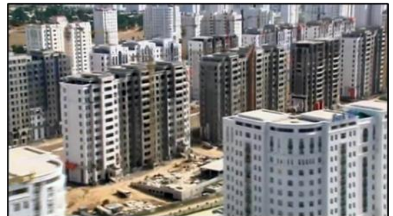
Figure 1. RC tunnel-form buildings in Ashgabat
